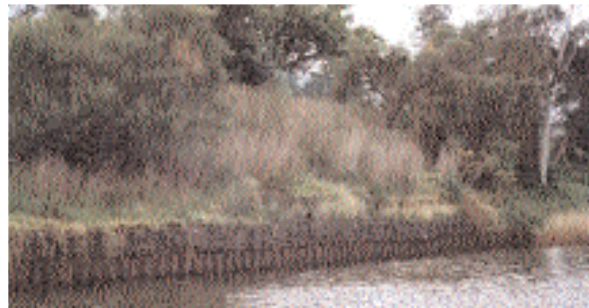
Erosion control structures such as sheet piling add little to the aesthetic value of the river and create long-term management problems.
